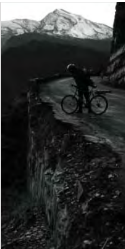
Fixing Going-to-the-Sun Road and increasing funding for park operations will protect a major economic asset
